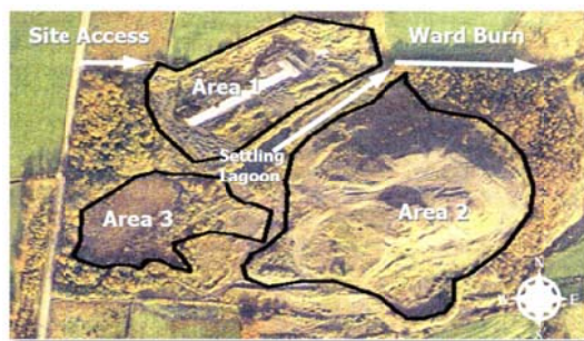
Figure 1: Site areas before redevelopment
