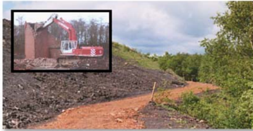
Figure 3: Demolition of Brickworks & Construction of Paths
